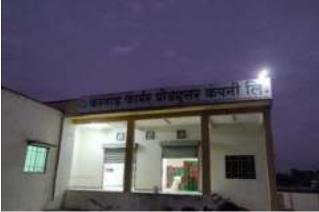
Export facility centre, Karmad
