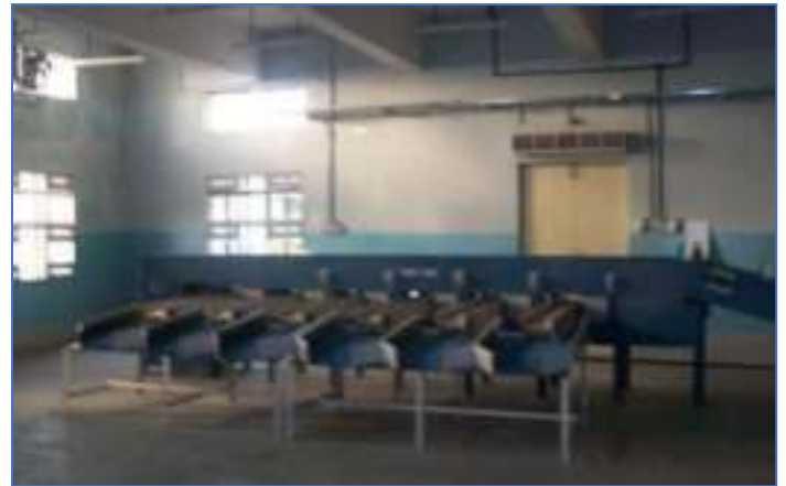
Grading lines Export facility centre, Jalna
