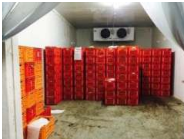
Cold storage Export facility centre, Ardhapur
