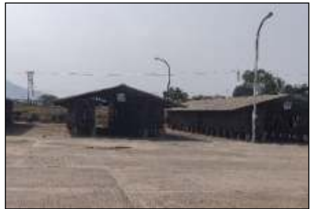
Figure 4.2.2: Onion storage, Export facility center, Kalvan
