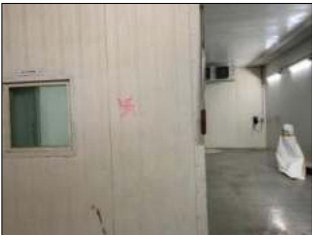
Cold storage, Export facility centre, Talegaon Dabhade
