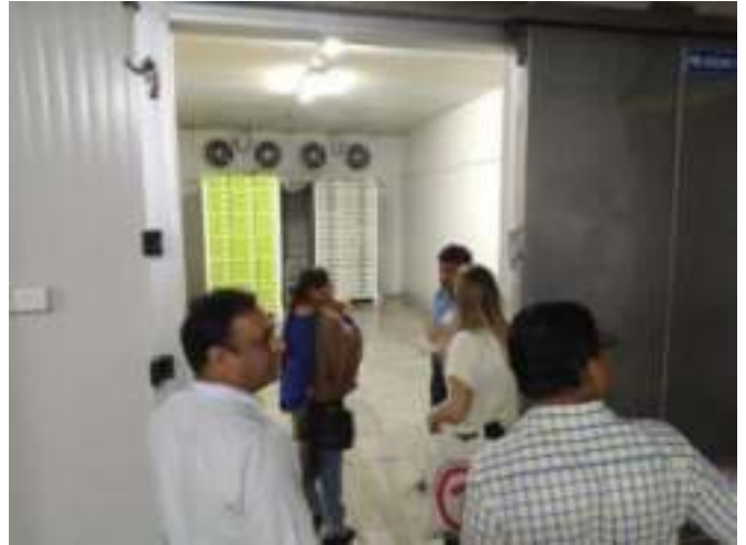
Figure 4.1.2: Cold storage, Export Facility Centre, Mohadi
